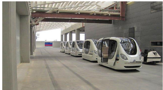
Figure 1. PRT system at Masdar.
